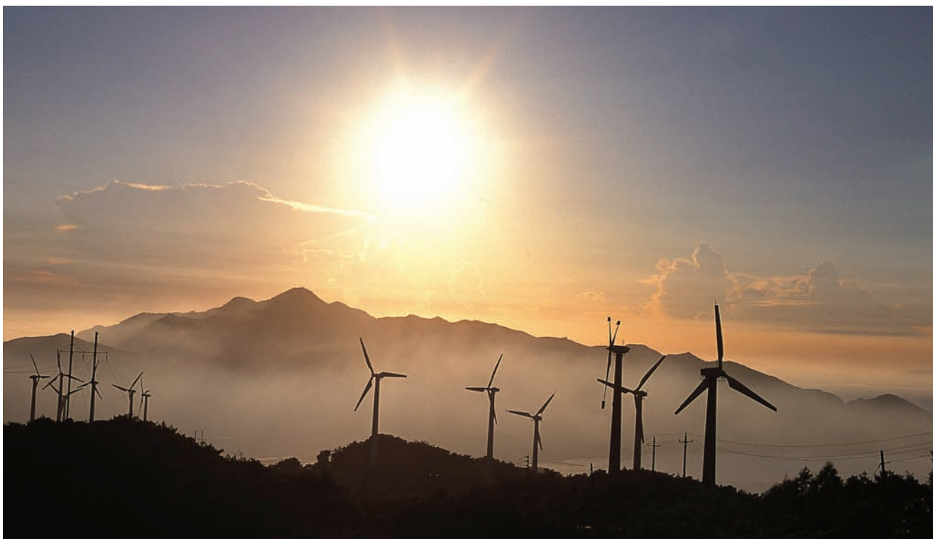
Wind farm in Guangdong Province, China. ©Greenpeace/Canxiong
