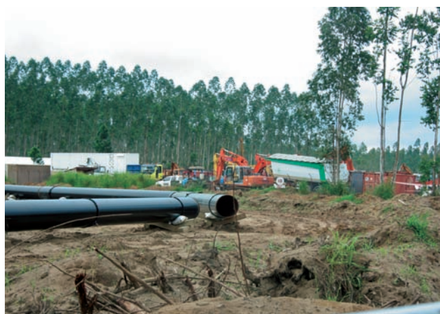
Building the new gas pipeline from M'Boundi to Djeno. © Elena Gerebizza
