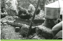
Inspection of the water channel that exits the 1.5 kW pelton micro-hydropower unit at Baan Naa Tam. www.palangthai.org
