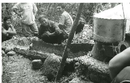
Inspection of the water channel that exits the 1.5 kW pelton micro-hydropower unit at Baan Naa Tam. [www.palangthai.org](http://www.palangthai.org)
