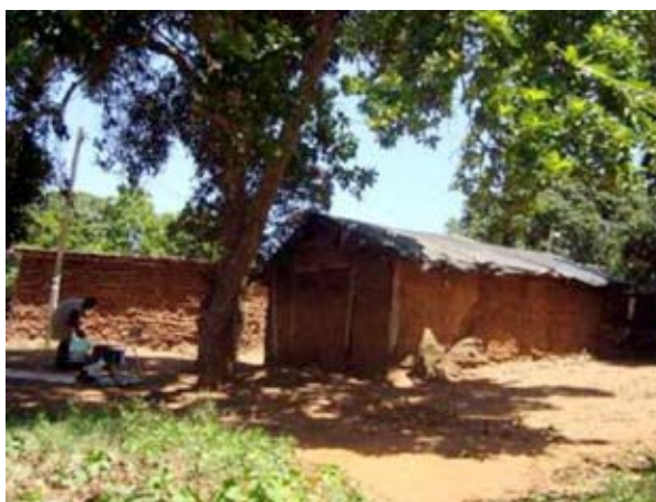
Figure 10: Mud House in Mkhwanazi Rural Community
