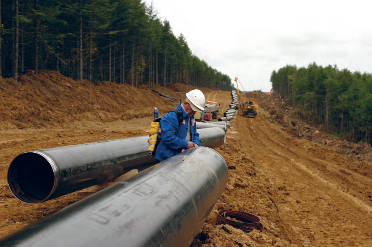
Pipeline-Bau in Russland. (© Peter Blakely – Redux/laif)
